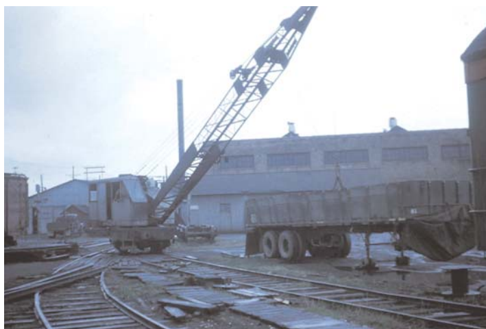
Pulling up rail prior to its delivery in Union.
